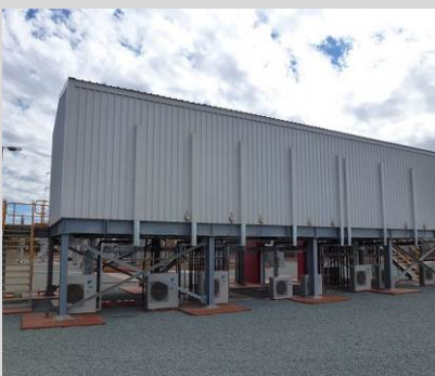
Substation Control Systems Commissioning
